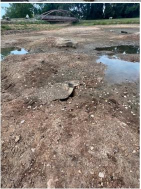
Paradise Lake in King Jack Park has been the subject of several conversations recently due to the loss of water again this year. Staff have put together a plan and an estimate of cost to try and seal the areas that are leaking up. The water is so low now that we plan to move a large amount of clay to the area and use a dozer to push and compact it over the areas of obvious leak occurring. Estimated cost to be \$12-\$15,000 subject to council approval.
