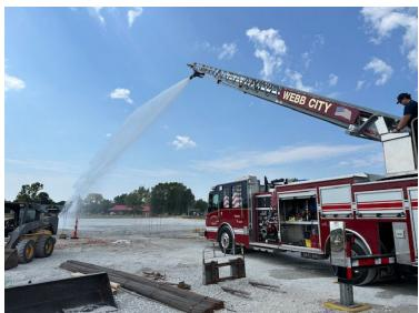
The new "W Club" Recreation area is moving along well. The Fire Department has been helping with the compaction of the pad by spraying water down which will help as they start the concrete pour. We should start to see the structure going up in the next week.
